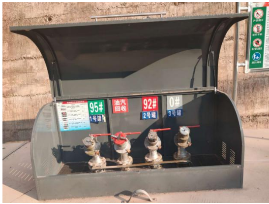
卸油口及卸油口油气回收
