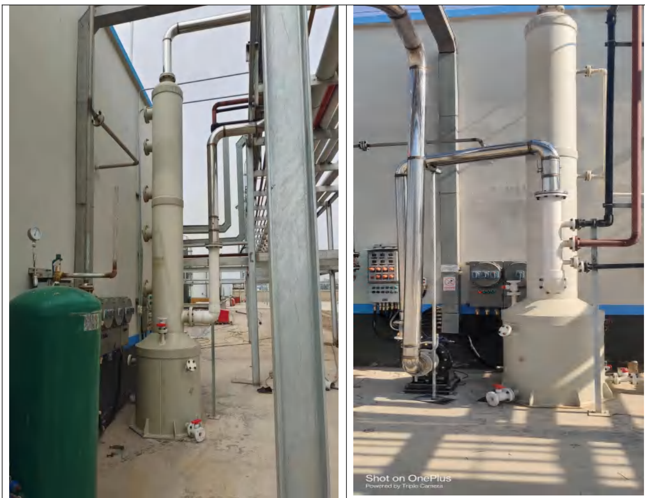
罐区碱喷淋塔喷淋
