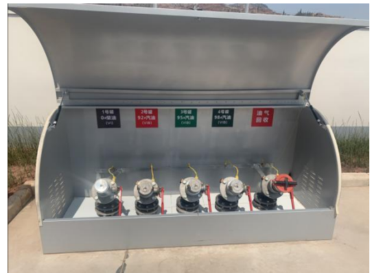
卸油口及卸油口油气回收
