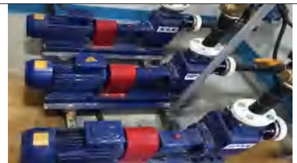
产水自吸泵、反洗自吸泵
